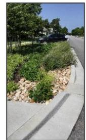
Parking lots can likewise be enhanced by use of **porous pavers** and bioswales for infiltrating rainfall in place of curb and gutter systems that otherwise discharge pollutants directly to adjacent streams. When properly designed and maintained, these **“green spaces”** can be an important amenity to residential and commercial properties.
